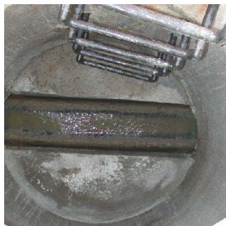
Manhole after restoration
