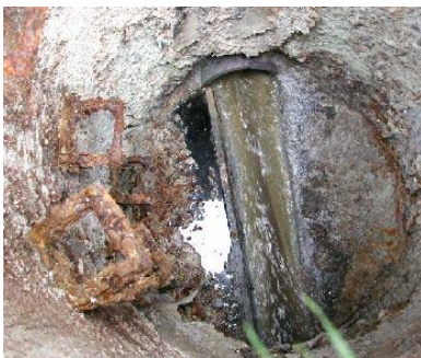
Manhole bevor restoration
